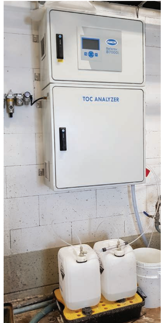
Installation of the TOC Analyser Hach BioTector B7000i at Steinbeis.
